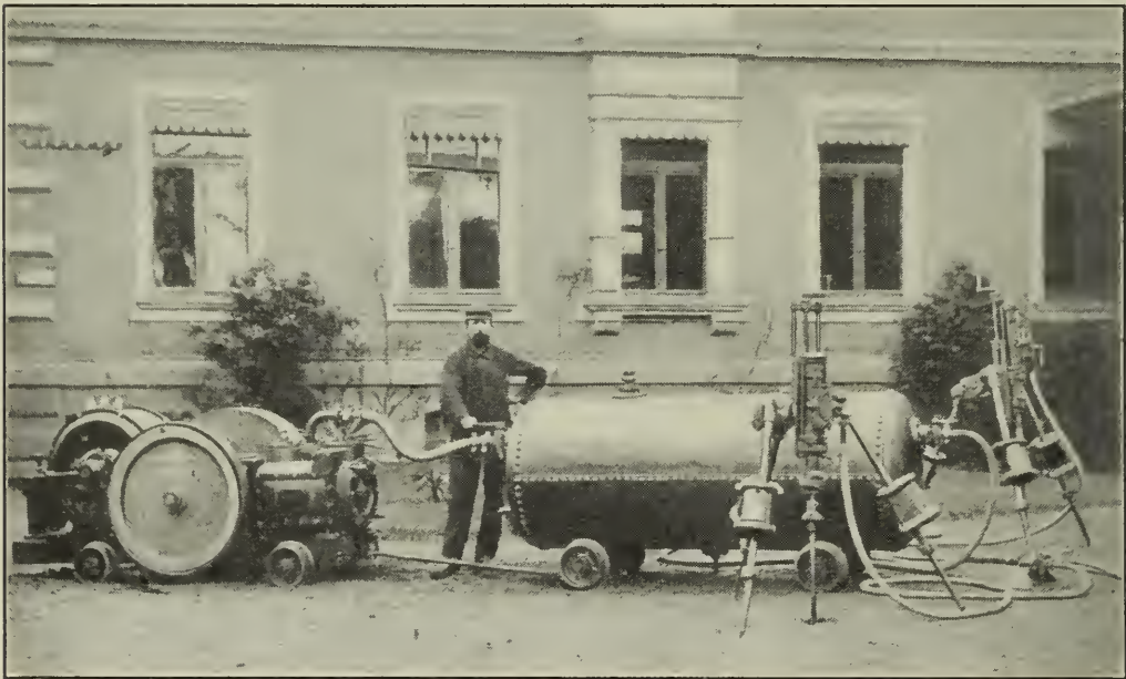
FIG. 19. ELECTRIC-DRIVEN AIR COMPRESSOR FOR MINING DRILL OUTFIT.
